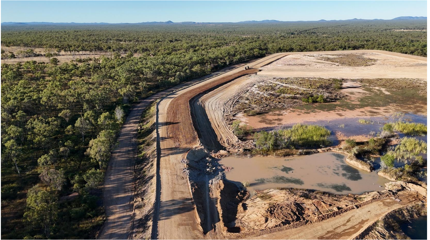
Figure 10: TSF temporary bund wall separating northern and southern cell
