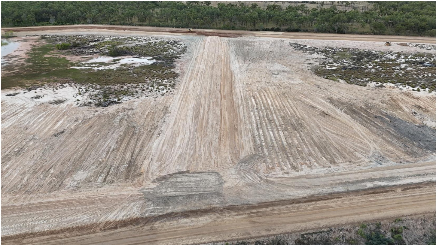
Figure 9: TSF temporary bund wall separating northern and southern cell
