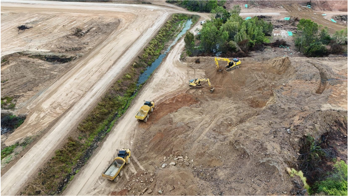
Figure 8: Mixing and blending of material for TSF embankment lift to crest height, supervised by ATC Williams
